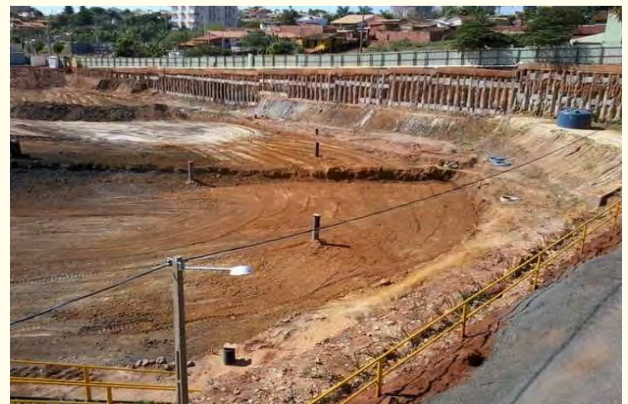
Figure 6: Situation after lowering system.
