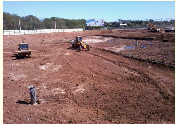
Figure 5: Situation after lowering system.
