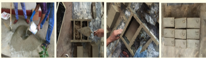
Figure 2: GSA-Cement block casting process.
